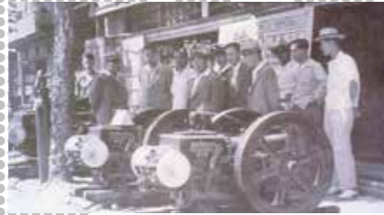
1956 Building of engines and diesel engines
